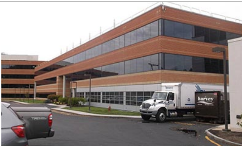
1 and 5 Mountain Rd., Framingham MA
